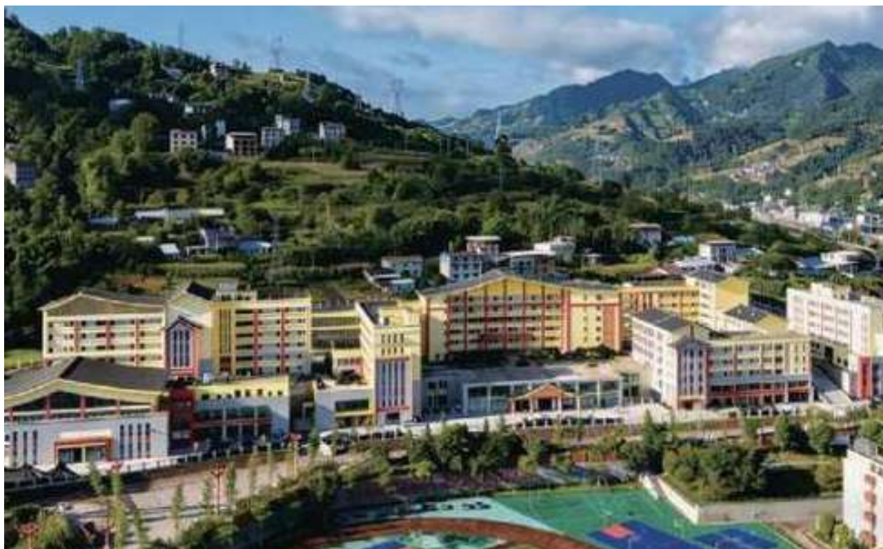
Pension finance: Sichuan Branch supported the Regional Elderly Care Center Project in Xiaoliangshan, Mabian Yi Autonomous County
