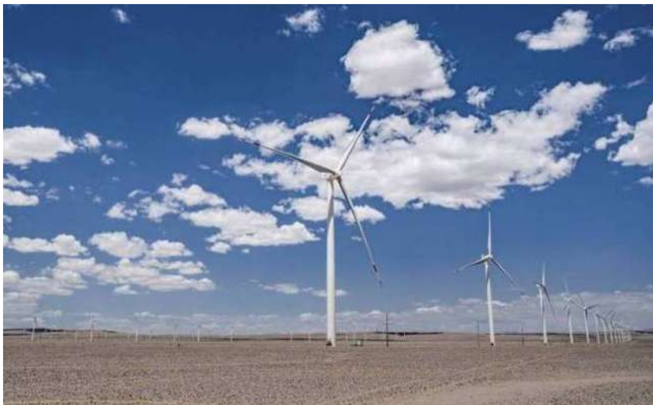
Green finance: Qinghai Branch supported the Wind Power Project at the Integrated Photovoltaic and Concentrated Solar Power Demonstration Base
